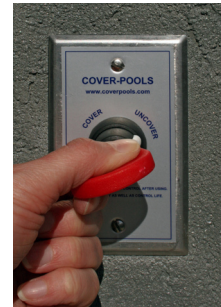
NEW: Hardwired control with key switch flush-mounted on wall (can be surface-mounted)
